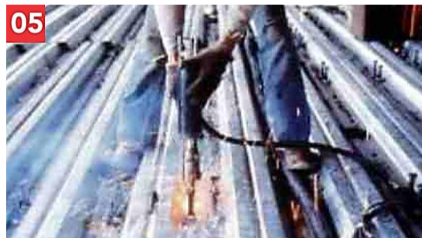
5 Fix SMARTDEK® to steel or concrete beam if required
