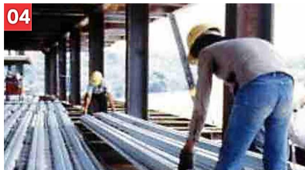
4 Place on steel or concrete beam
